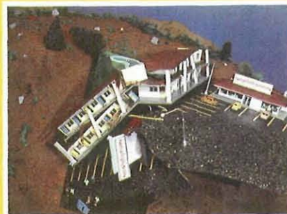
EDIFICE WRECK—San Andreas, California "It's not our fault."
